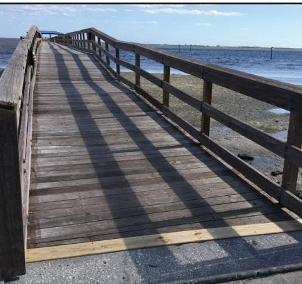
In November 2020, Hurricane ETA damaged a portion of the pier at Safety Harbor Marina. Engineering coordinated with Augustine Construction to perform immediate repairs of the damaged railing, stringers, and decking for approximately **40** feet starting at the entrance of the Pier. Repairs were completed in two days.
