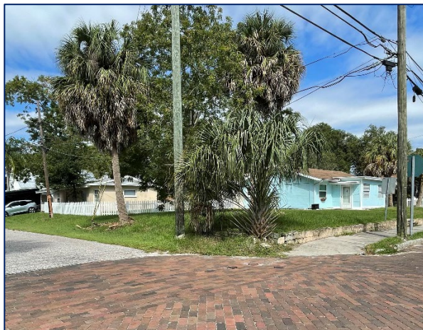
Intersection without curb ramp and detectable warnings
