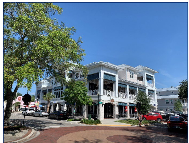
Recent Intersection Improvements on Main Street
